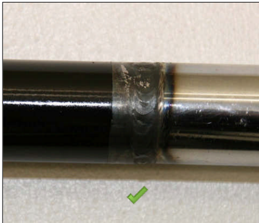
Picture of Acceptable Permanent Weld
